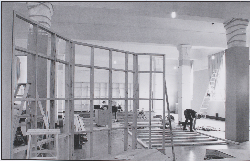
Construction underway on the first floor developments.
