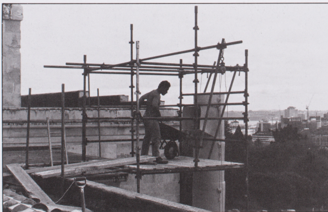
Repairs to Museum roof, photographed by Virginia Bennett
