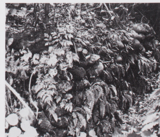
At Kōru old stone work which holds up the steep scarps can still be seen beneath ferns and other native plants.
