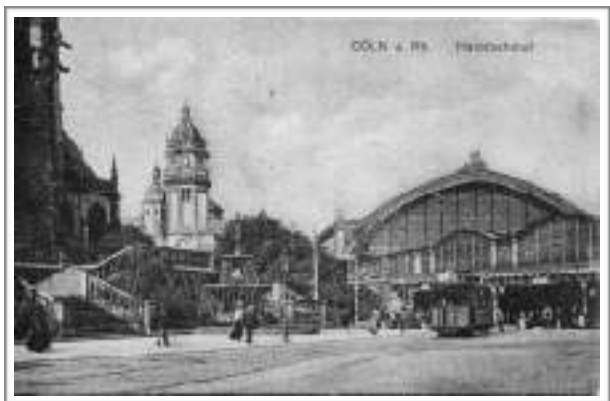
This is part of the railway station just over the large bridges. With love Jamie
