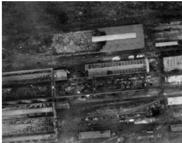
Low-level photographic reconnaissance photograph of blast-damaged buildings at the Breuil steelworks at Le Creusot, France, following the special low-level daylight raid by Avro Lancasters of No. 5 Group, Bomber Command, on 17 October 1942. From: bomber-commands-operation-robinson-hits-le-creusot-works#sthash.bSvjZMLu.dpuf
