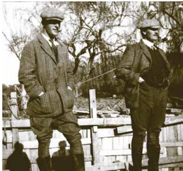
Poppa, land drainage engineer in local charge of the Rangitaiki works, with JB Thompson, Chief Drainage Engineer, c. 1912. Owen would succeed Thompson in 1922 when Thompson became Under-Secretary of Lands.
