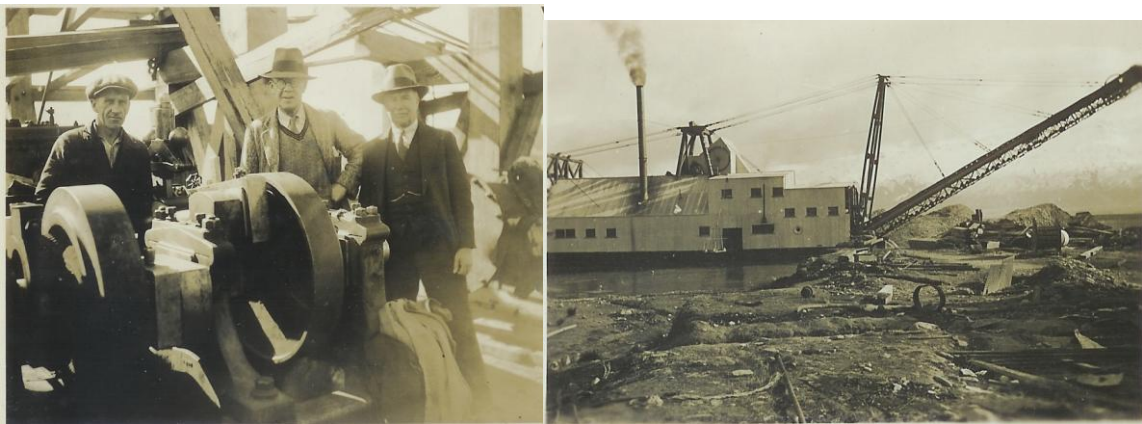
Installing the engine for the "Goldlights" dredge. "Goldlights" dredge working at Bendigo Creek George McKnight on left
